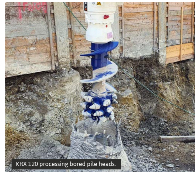
KRX 110 cutting bored piles.
