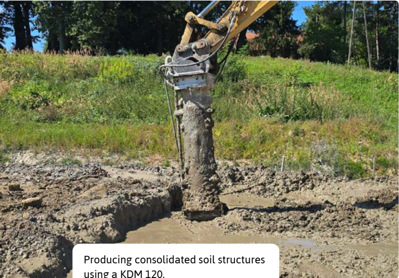
Cured and profiled soil block that was installed with a KDM 120.
